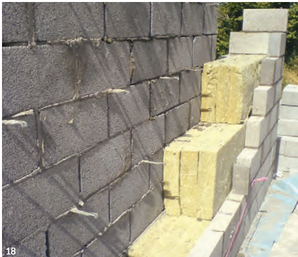
Below: The home has super insulated thermally massive construction, a large south facing sunspace and a monopitch, south east facing roof
